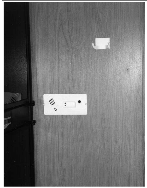
Fig. 6-4 CARBON MONOXIDE MONITOR
