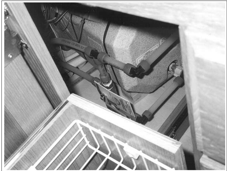
Fig. 4-19 WATER HEATER DIVERTER VALVE
