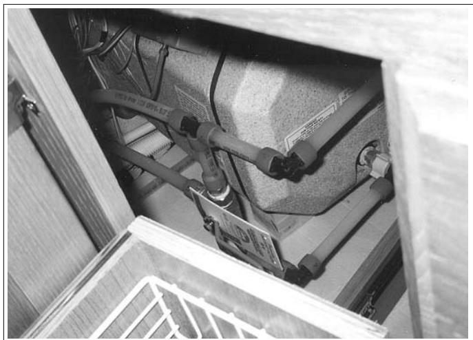
Fig. 13-7 BYPASS VALVE
