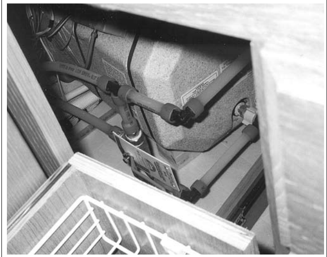
Fig. 17-1 BYPASS VALVE
