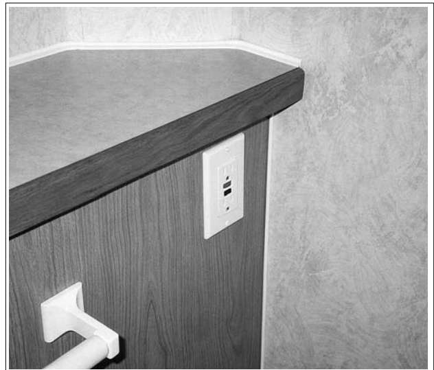
Fig. 10-5 GFCI OUTLET (TYPICAL)
