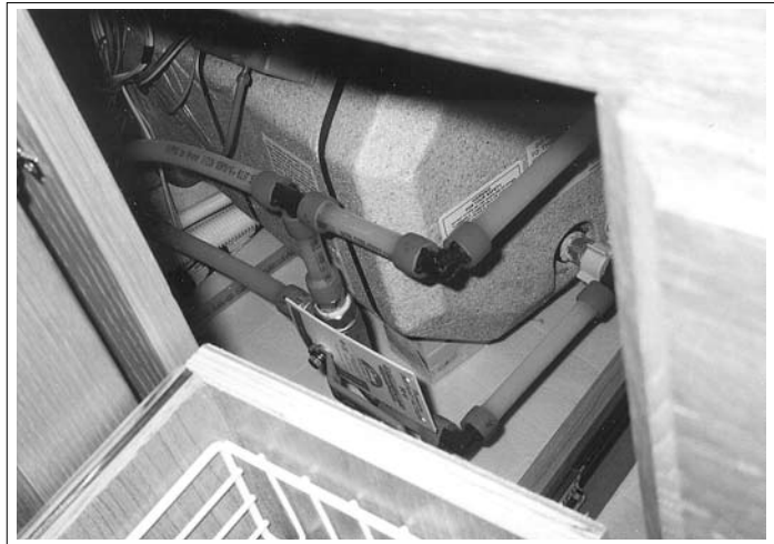
Fig. 12-7 BYPASS VALVE
