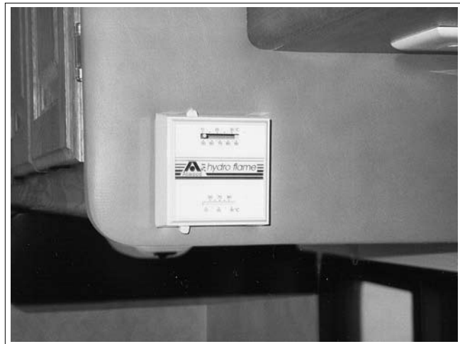
Fig. 13-8 FURNACE CONTROLS
